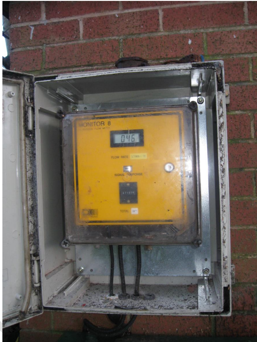
Discharge Pumping Chamber No 2 Flowmeter
