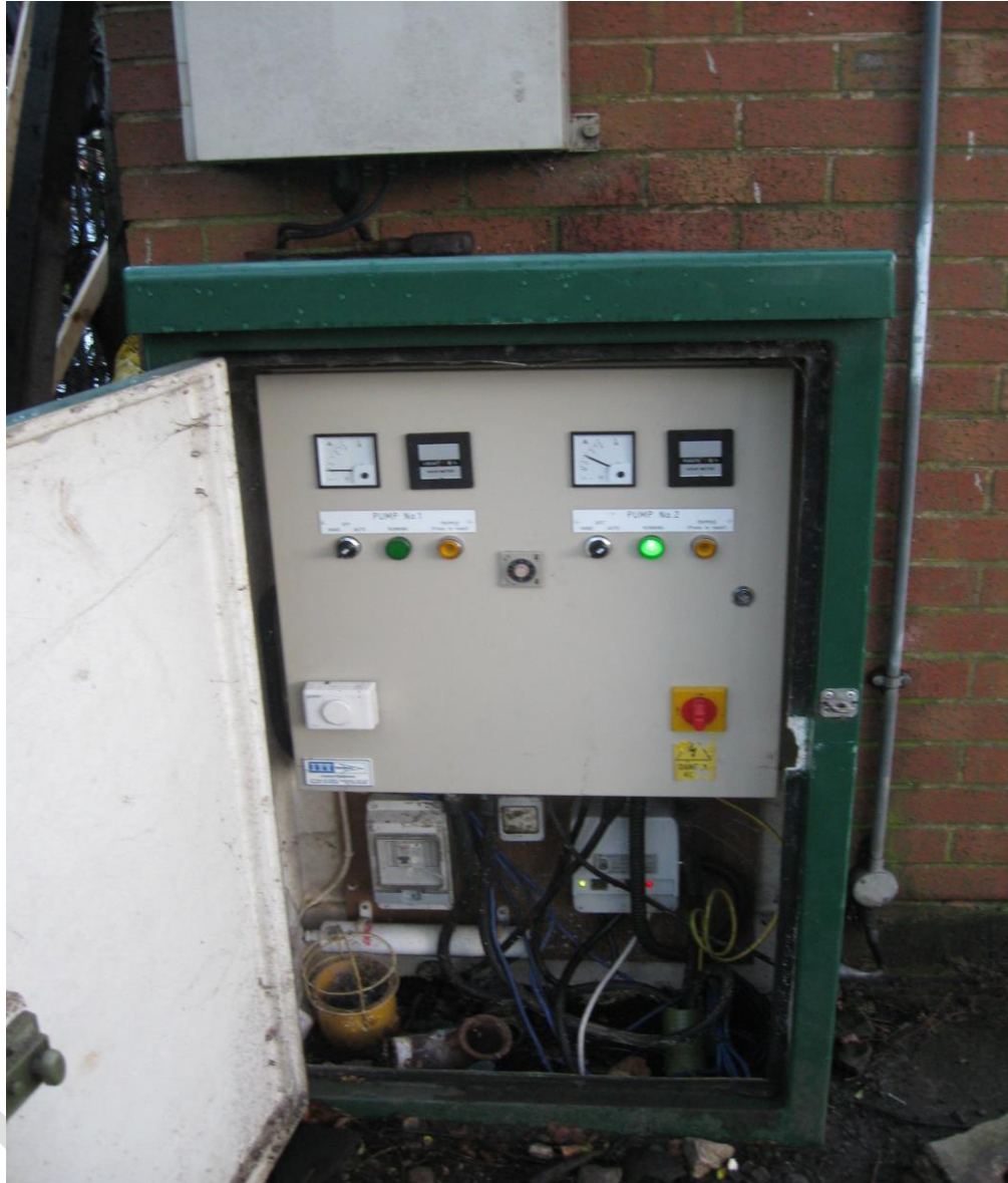
Discharge Pumping Chamber No 2 Control Panel
