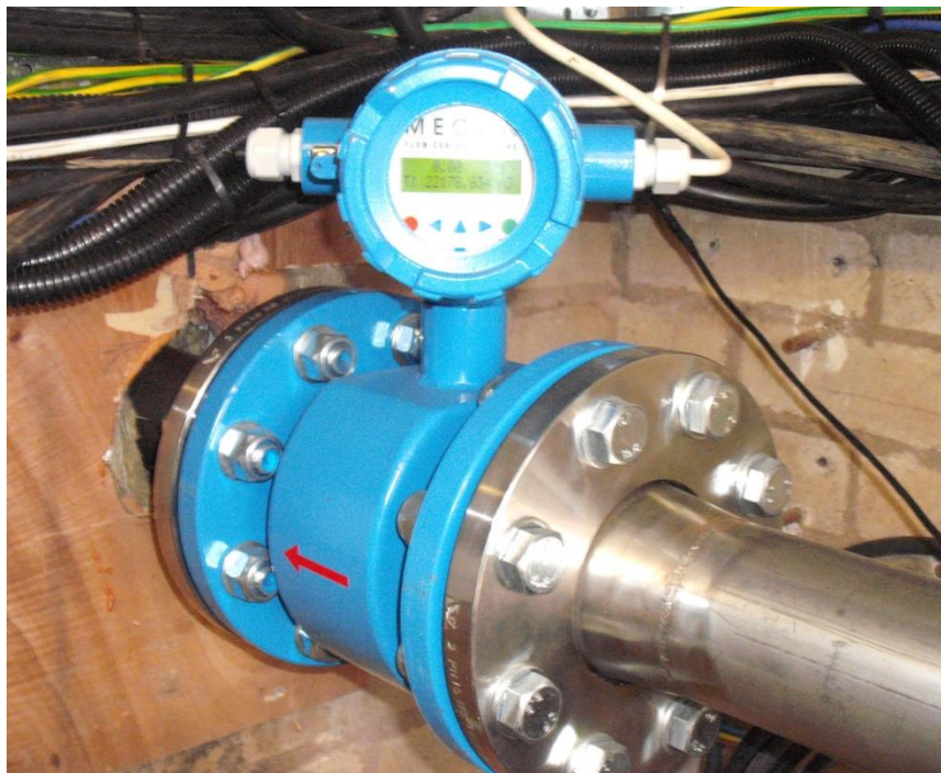
Flow meter and display panel
