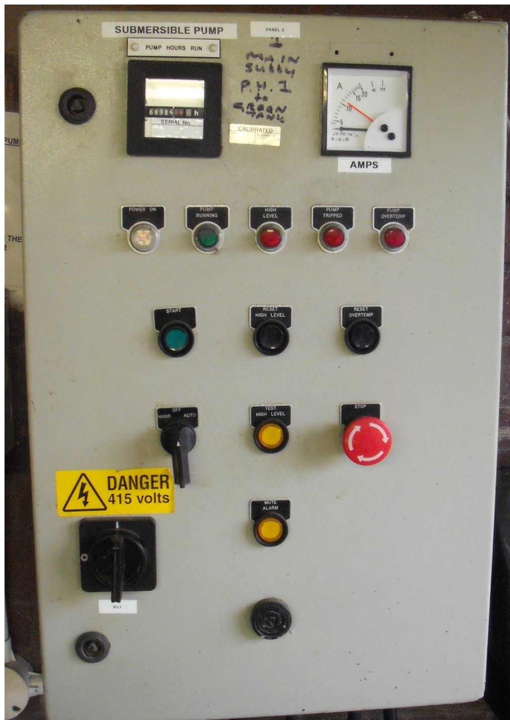
Submersible (Supply) pump control panel
