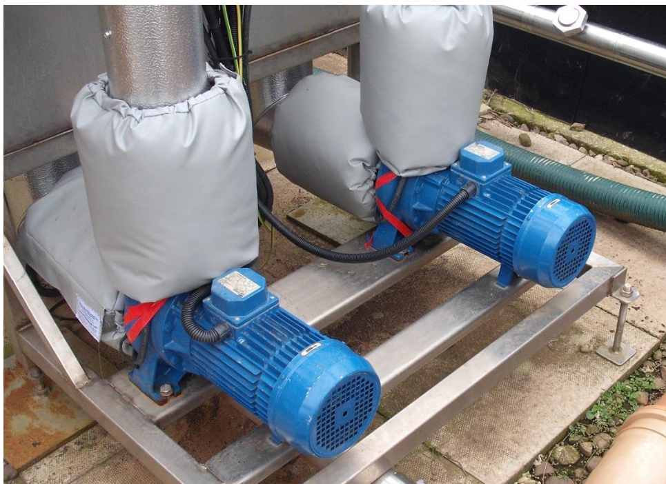
Centrifugal (Transfer) Pumps mounted onto Sparge tank
