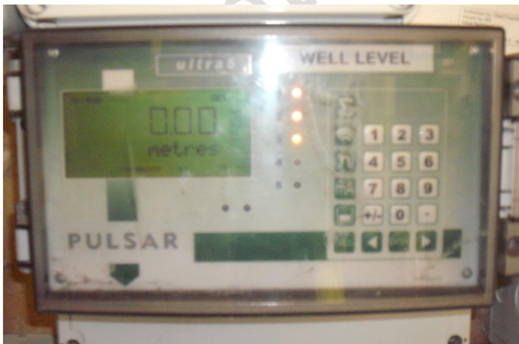
Telemetry display panel
