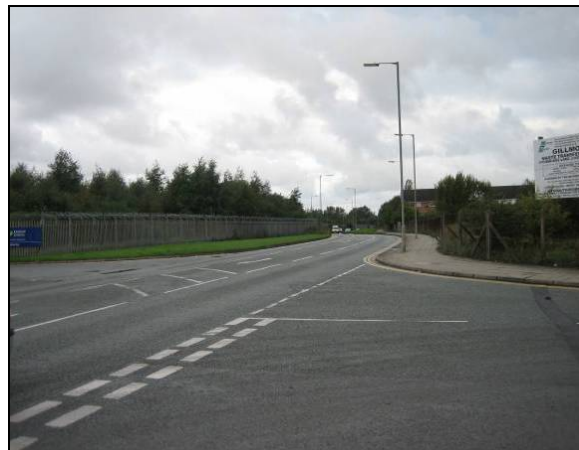
Figure 5.1 – Stonebridge Lane Looking North (Taken 04/10/06 08:05 am)
