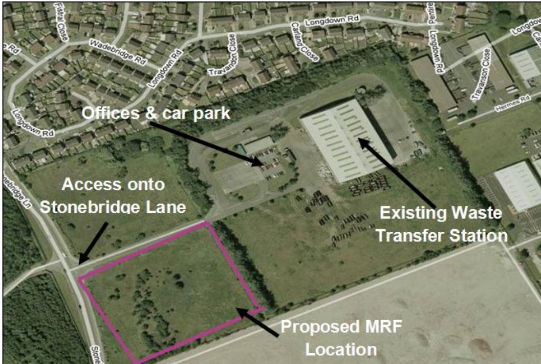
Figure 3.1 – Aerial Photo Showing Site Layout
