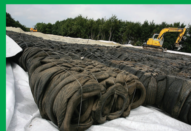
Baled tyres being re-used as road foundations
