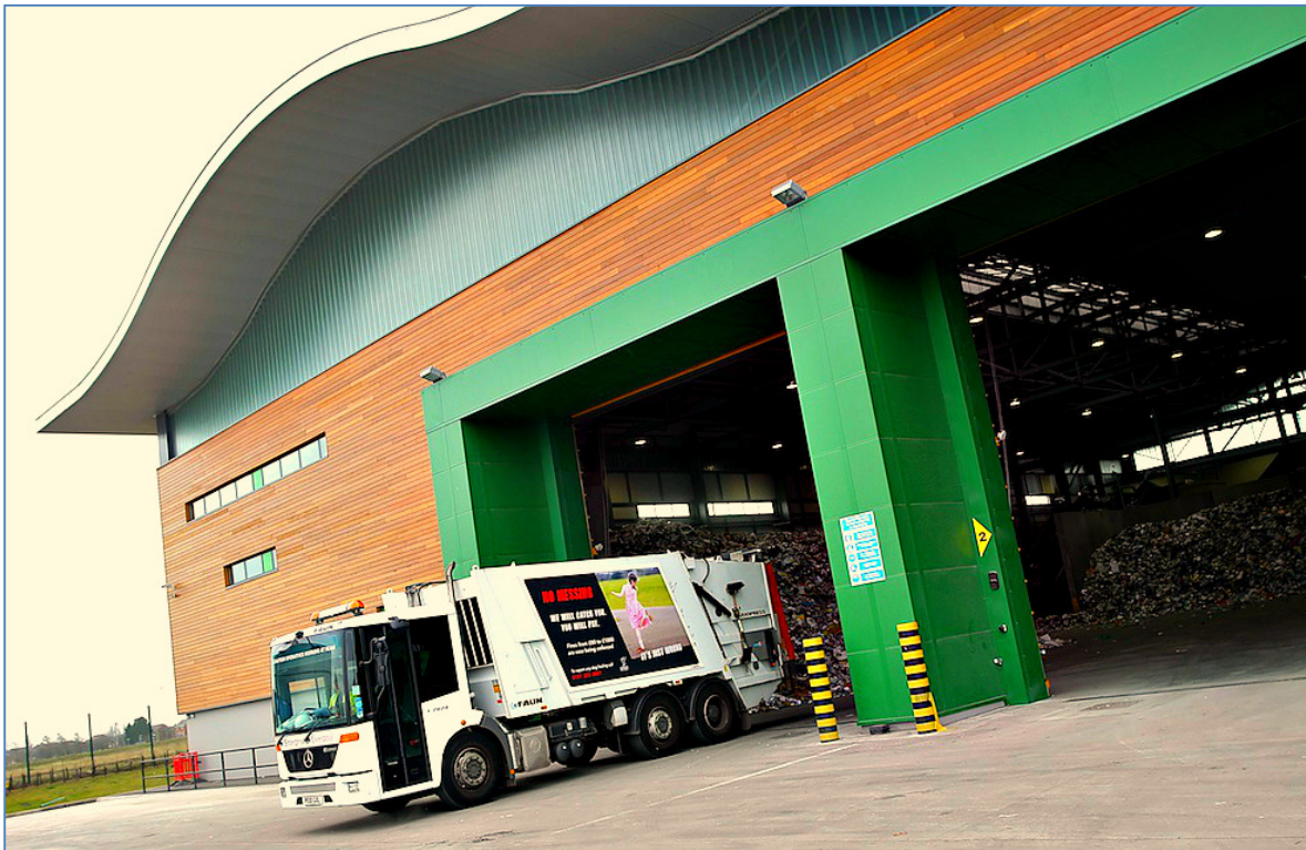
(Gillmoss Materials Recovery Facility)
